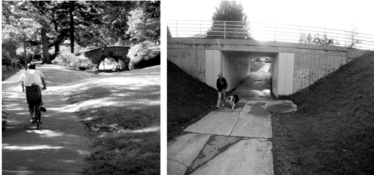
Figure 3. Radburn’s famous pedestrian underpass, a tunnel under Howard Avenue which connects Park A and Park B, Radburn’s two superblocks (left) and a pedestrian underpass connecting superblocks at Kitimat (right). Photos by the author.
