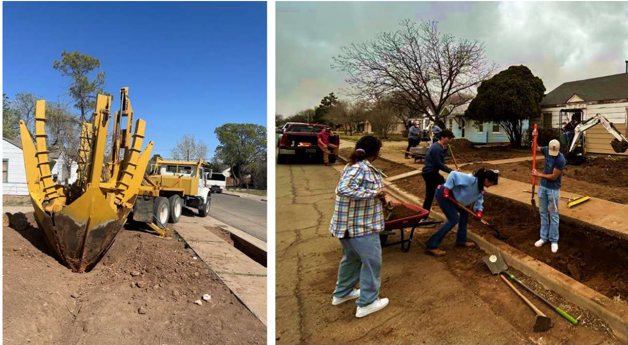
Figure 5. Translocation of mature trees was facilitated by truck-mounted tree spades (left) on loan from Texas Tech University. Students prepared sites using hand tools and mini excavators to increase the stormwater storage capacity of residential sites (right). Interventions included engagement with and excavation of median strips as a transitional zone between private and public space. PHOTOS: The Author
