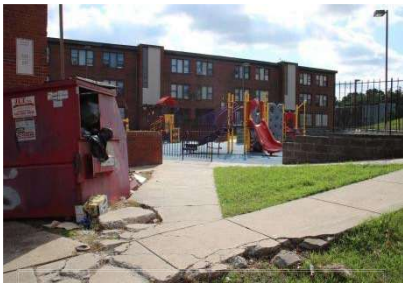
Figure 1. Damaged sidewalks and waste disposal along children's playground. Photo by the authors.
