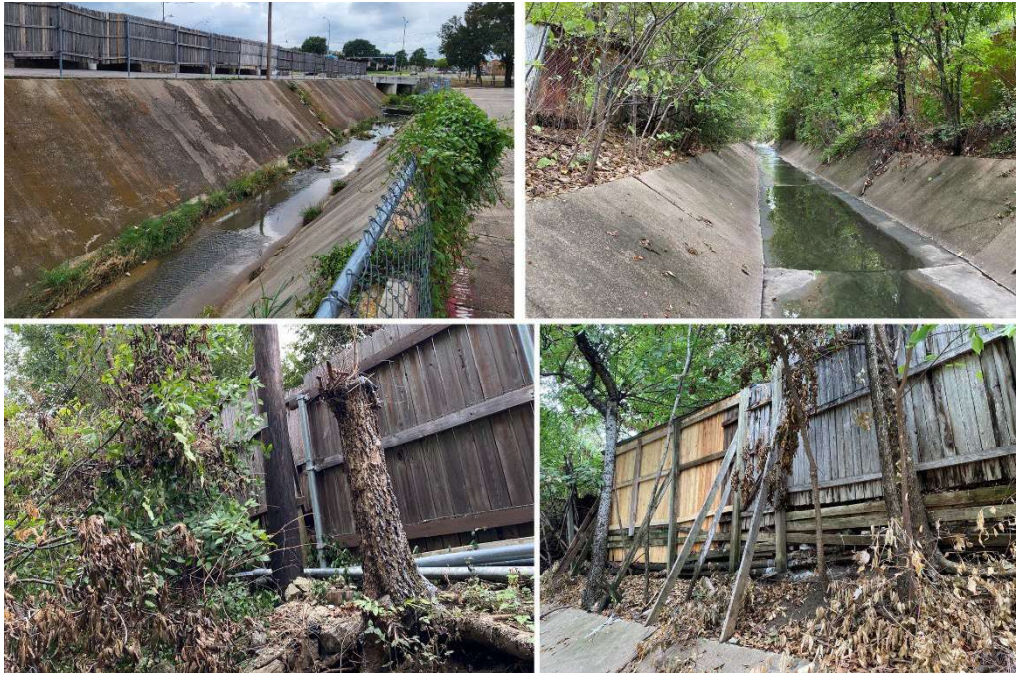
Figure 5. Site photos of channelized area in residential backyards.
