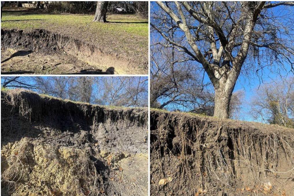
Figure 4. Site photos of erosion along the creek from adjacent neighborhoods.
