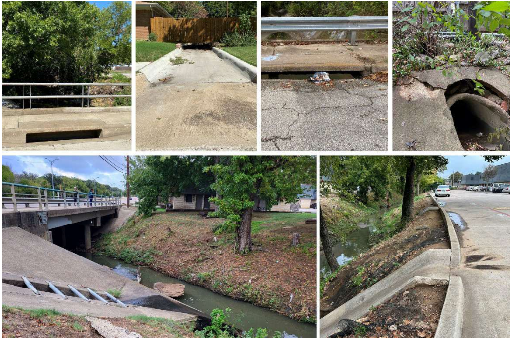
Figure 3. Site photos of drainage into the creek from adjacent roadways and neighborhoods.
