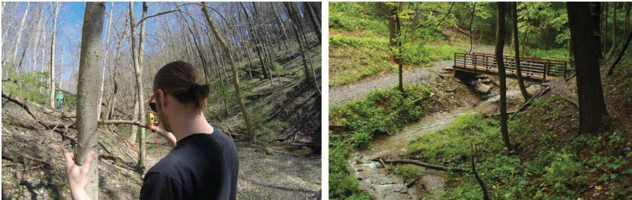
**Figure 4: Students measuring slope (with a clinometer) while flagging trails at Falling Run in 2016 compared to the nearly the same area as built in Sept. 2018. Photographs by author; students completed a media release.**
